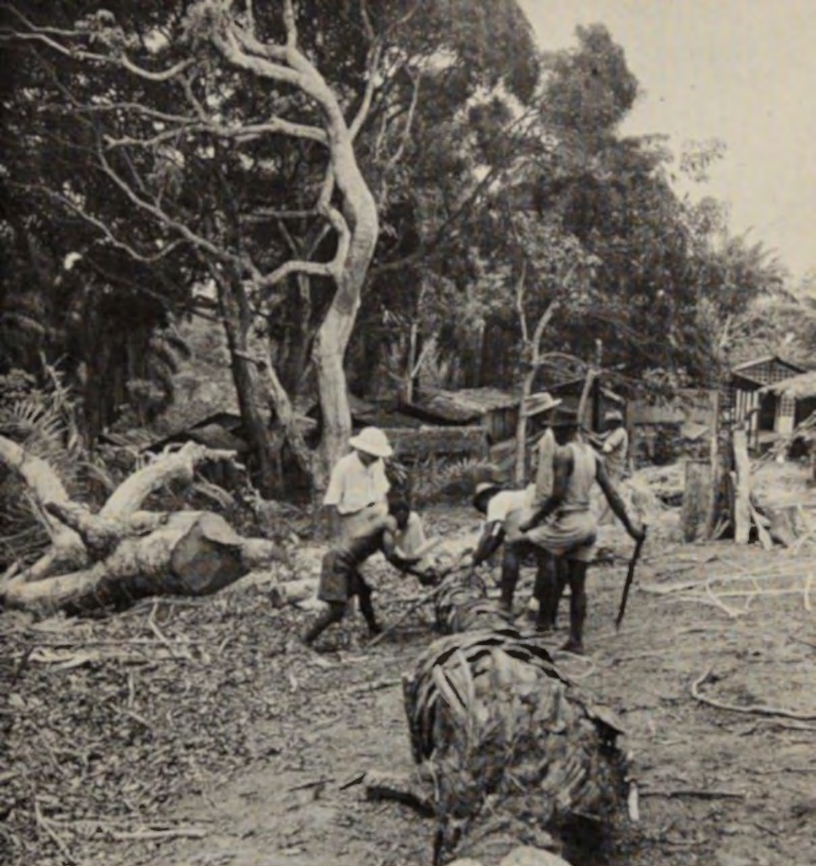
CLEARING GROUND FOR LEPER VILLAGE
